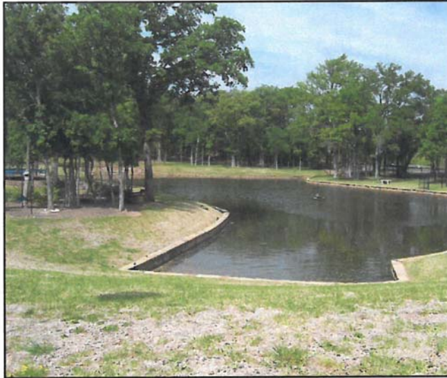
Figure 1: Retention Pond with Hardedge.
